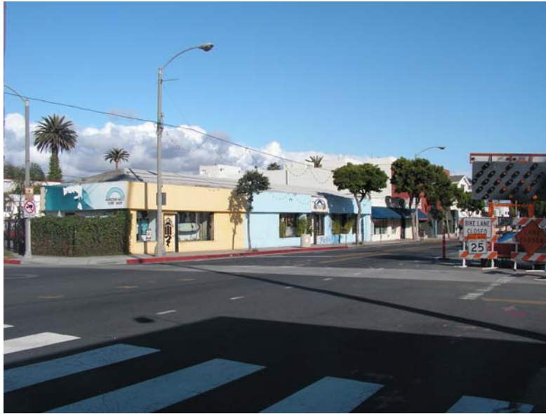
General View, 2001-2003 Main Street, View to Southeast.
